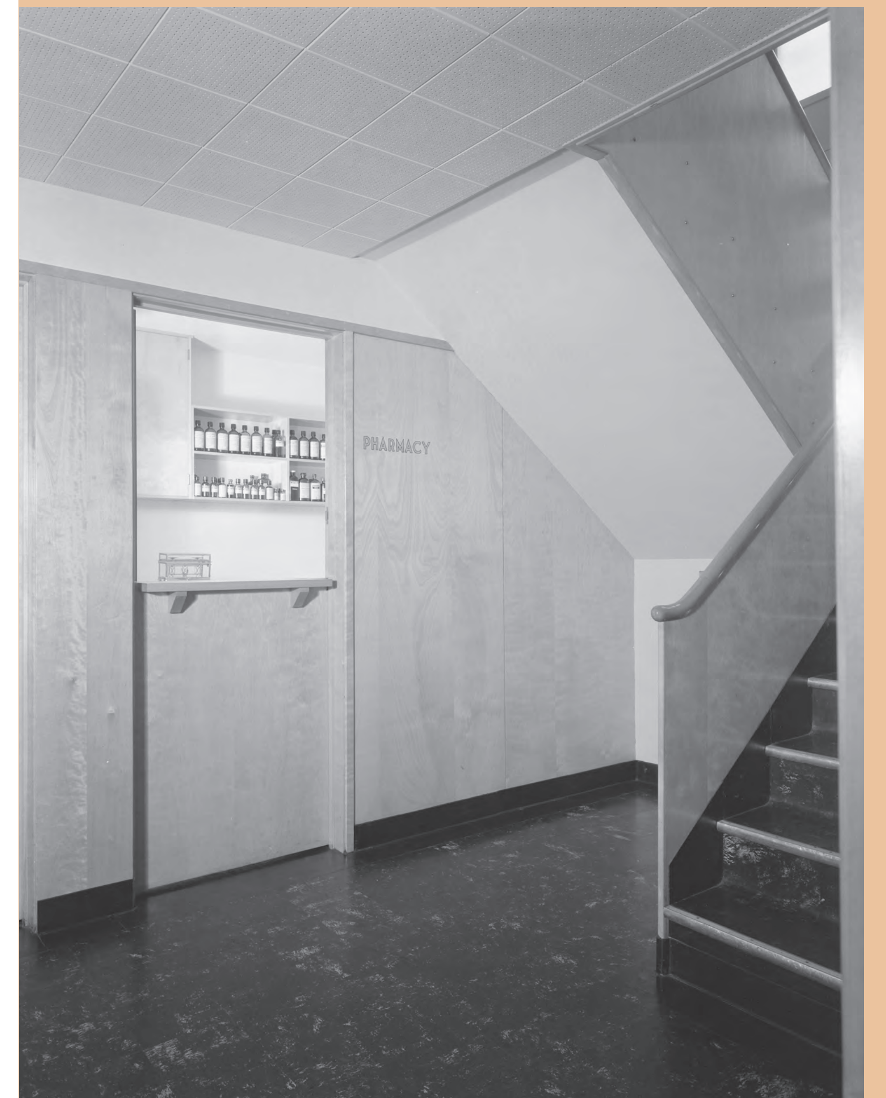
Close and Scheu used birch plywood throughout the building to handsome effect, including for the stair rail and pharmacy walls. HB-06586-P, Chicago History Museum, Hedrich-Blessing Collection.
