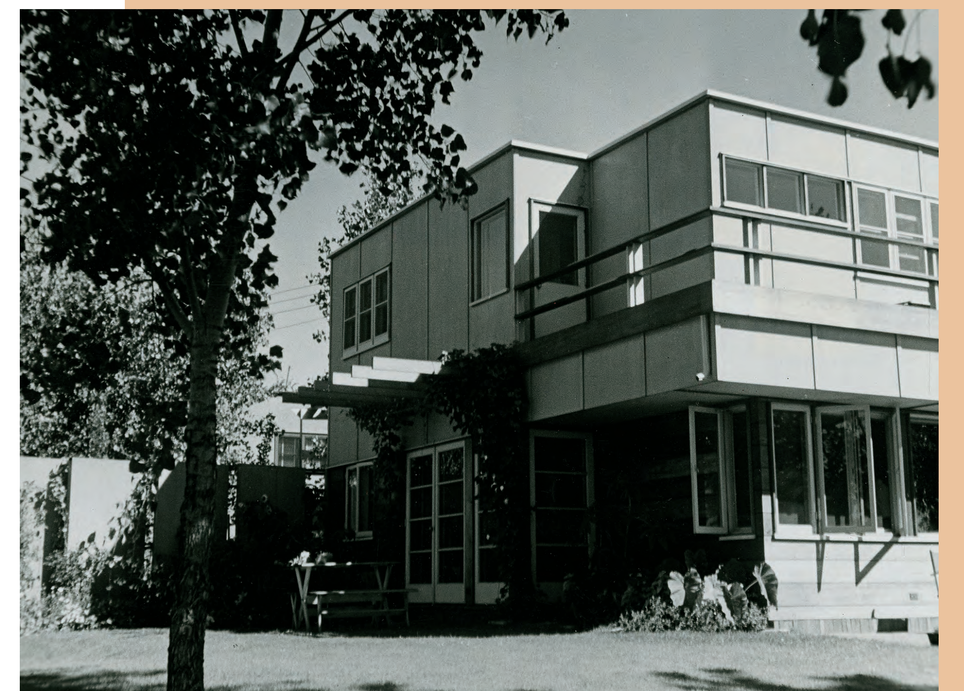
To complement the simple geometric forms of the Faulkner House, the architects specified durable, unfussy construction materials, including redwood siding and resin-bonded plywood. Close Associates Papers (N78), Northwest Architectural Archives, University of Minnesota Libraries, Minneapolis.
