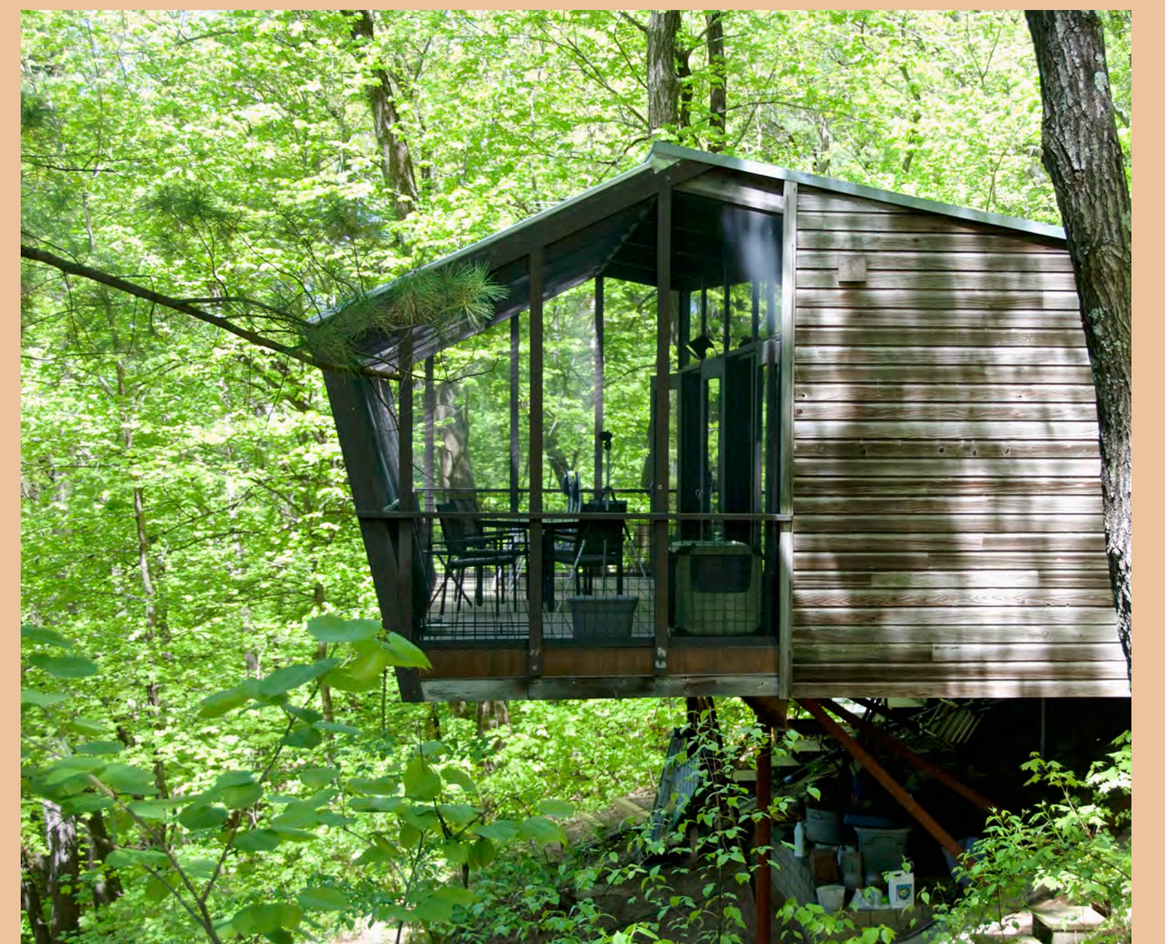
The second Skywater cabin (1961), built as a guesthouse, projects out from the hillside. Photograph by Jane King Hession.
