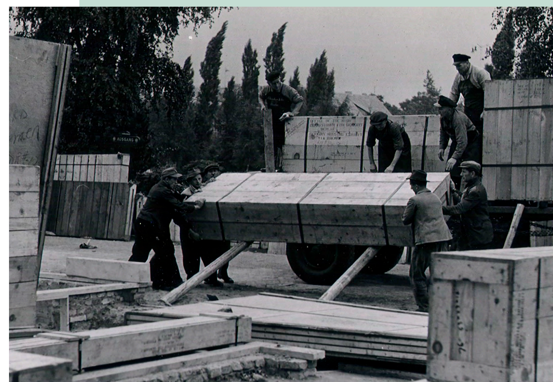
In 1950, the U.S. State Department shipped a "Jubilaire" Page & Hill house from Minnesota to Cold War Berlin to serve as the "Model American Home" at the German International Industrial Exhibition. Here, workers in Berlin unload boxes containing prefabricated sections of the house. National Archives, Text Division, RG59, 862A.191, box 5225.
