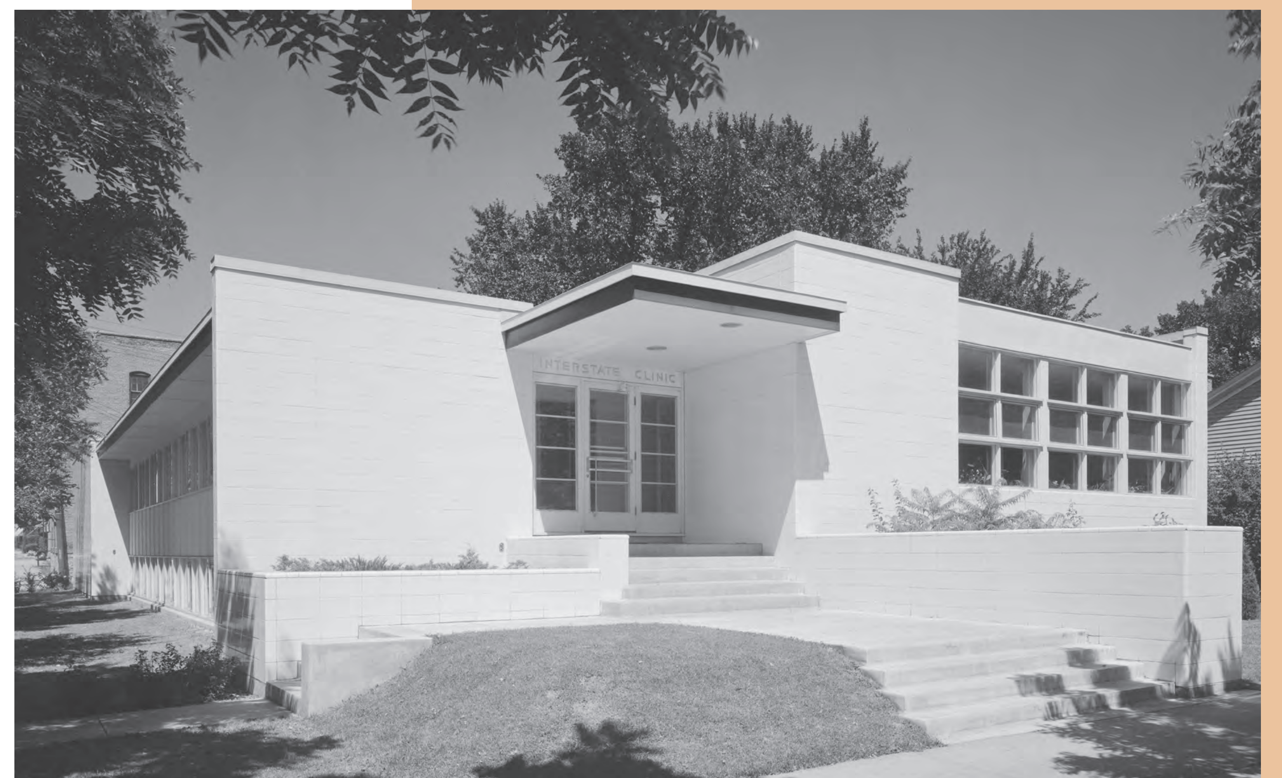
Glazed white tiles sheathed the simple, geometric volumes of the building. HB-06586-A, Chicago History Museum, Hedrich-Blessing Collection.
