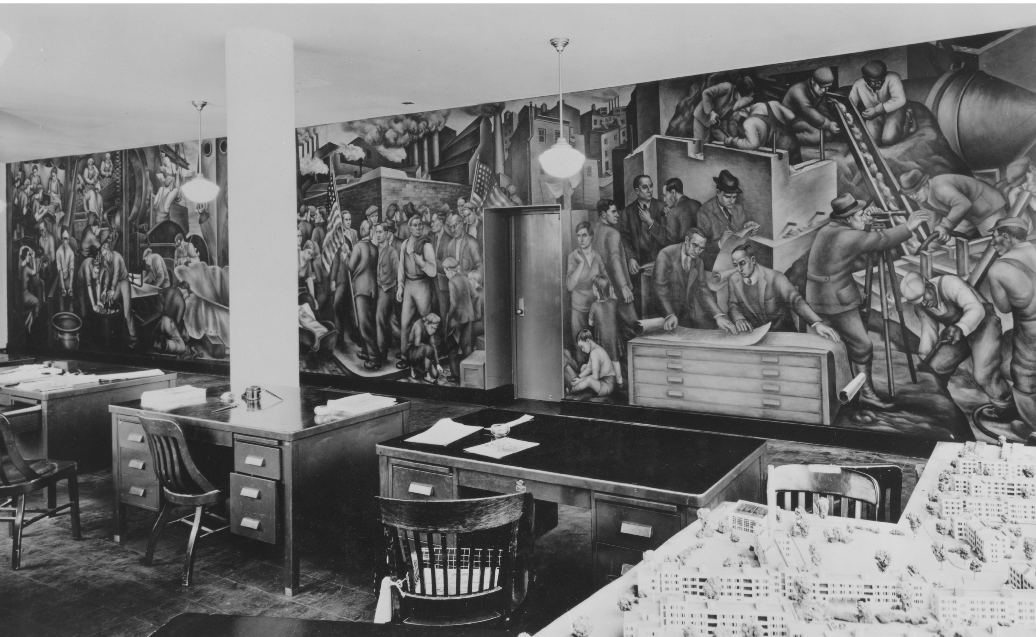
For Oskar Stonorov, Lisl worked on Westfield Acres (1938) in Camden, New Jersey, a PWA-sponsored project. In this photograph of the social room, a model of Westfield Acres can be seen at right. American muralist Marion Greenwood painted the labor-inspired scene on the wall. Westfield Acres Housing Project Social Room Murals, Camden, New Jersey, 1935–43; Treasury Relief Art Project: Missouri, New Mexico, New Jersey, New York; Records of the Public Buildings Service, Record Group 121; National Archives at College Park, College Park, Maryland.
