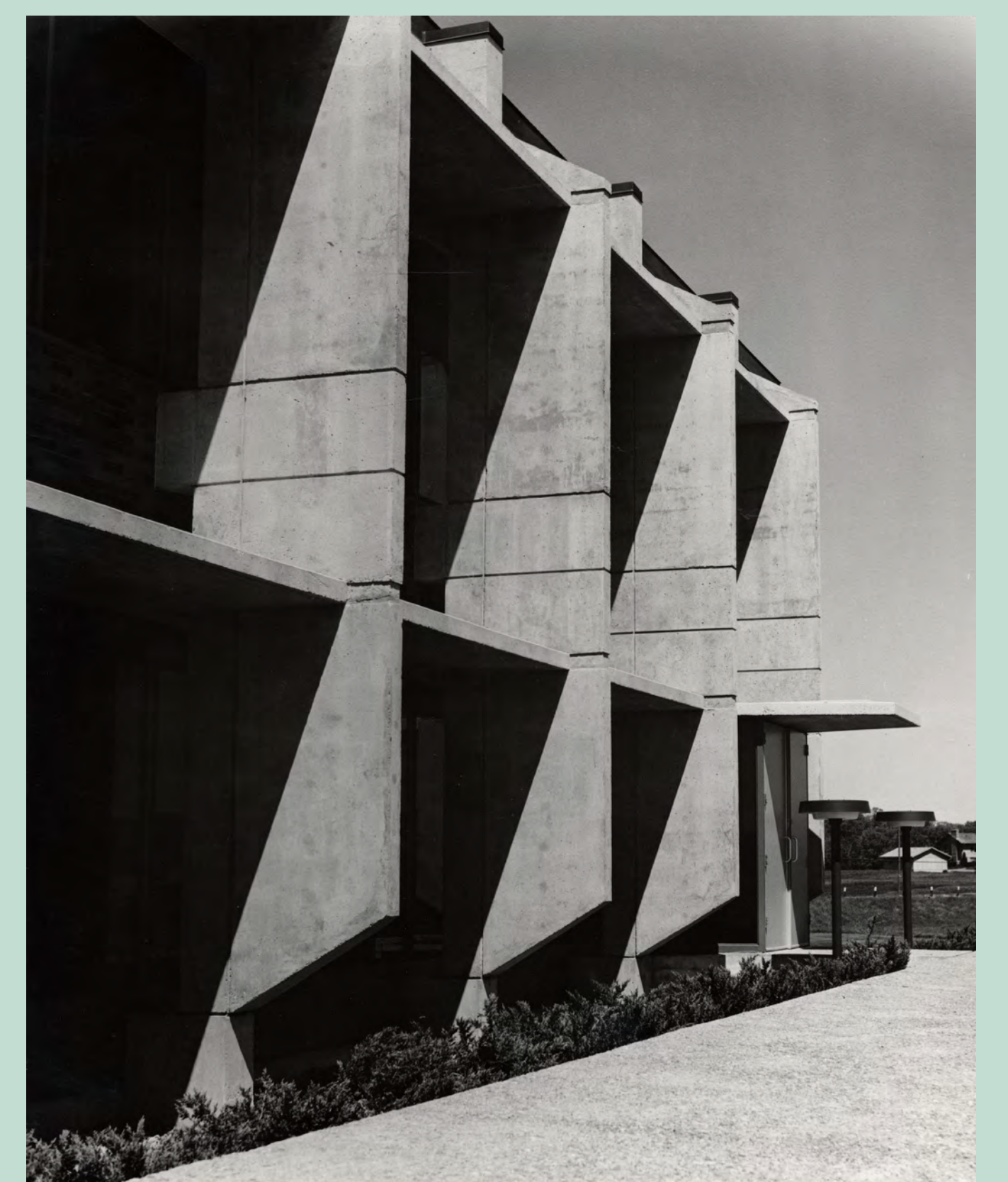
Concrete fins function as shading devices to protect interior spaces from excess sunlight. Photograph by Phillip MacMillan James & Associates. Close Associates Papers (N78), Northwest Architectural Archives, University of Minnesota Libraries, Minneapolis.
