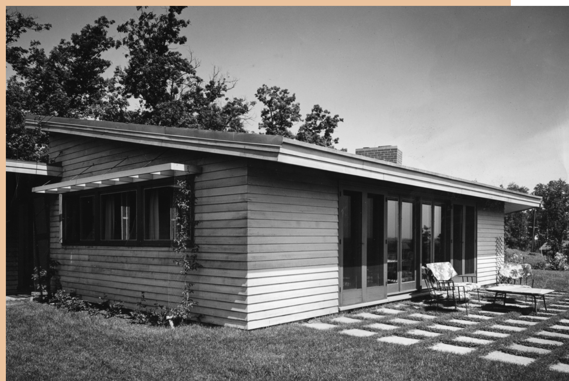
The Dr. Ruth Boynton and Prudence Cutright House (1948) in Bloomington, Minnesota. Photograph by Lucian H. Brown. Close Associates Papers (N78), Northwest Architectural Archives, University of Minnesota Libraries, Minneapolis.
