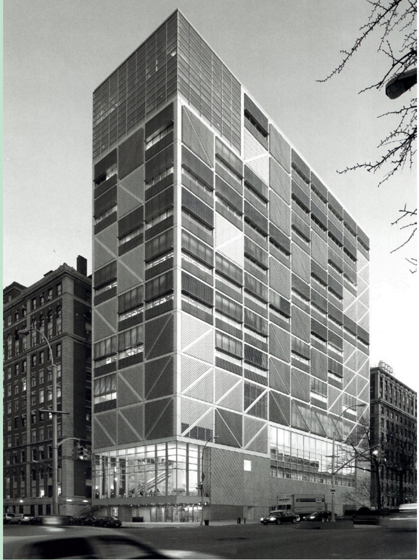
Figura 1: Moneo NorthWest Corner Building Columbia University, NY
